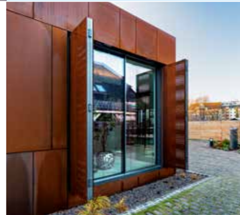
Sliding folding shutters made of Corten steel. Slat sun protection for historic buildings.
